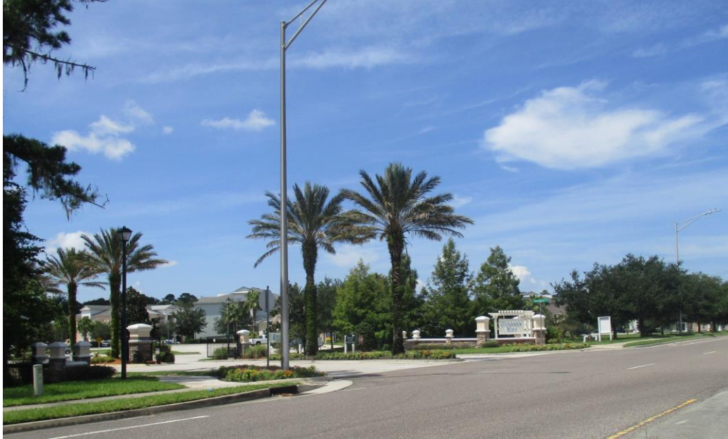
Condominiums to the east along A C Skinner Parkway (4916 Sunset Marina Drive): Summer Key Condominiums
